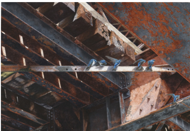
17x22 10-0072AW Bridge #1356
